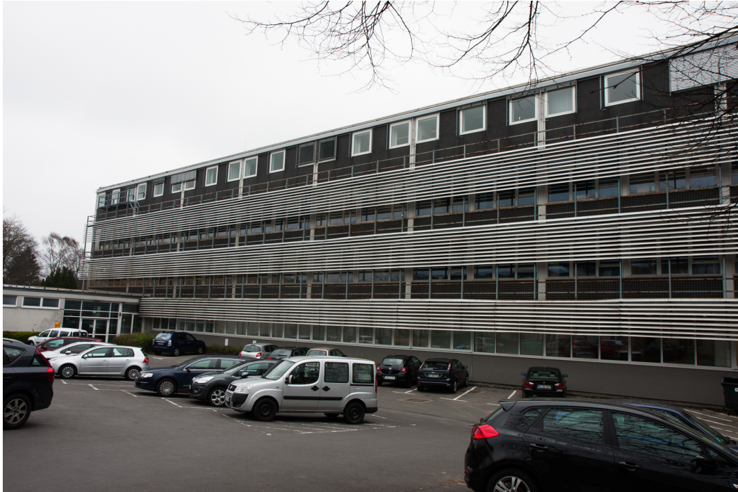
Figure 1.4: The iWall is installed at the third floor inside the sun blades of the historical computer science building.
